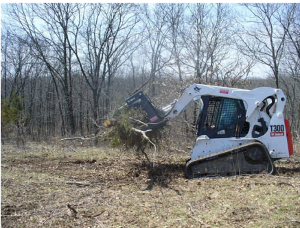
A Midwest Land Restoration crew clearing the site of debris.
